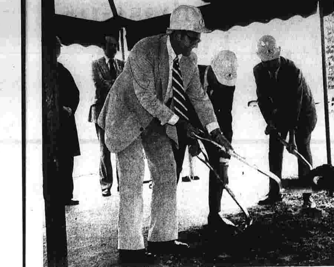
Donald Caldwell, president of the Board of Trustees of Rockville General Hospital, front left, turns a shovel of earth at ground-breaking ceremonies Wednesday for the $2.1 million addition to the hospital. Assisting him are Everett Paluska, Ellington's first selectman, center, and Mayor Frank McCoy of Vernon. Standing in the rear is the Rev. John White of St. Bernard's Church (behind post) and Chester Morgan, Vernon's state representative. Several other dignitaries attended the ceremony. (Herald photo by Antio)
